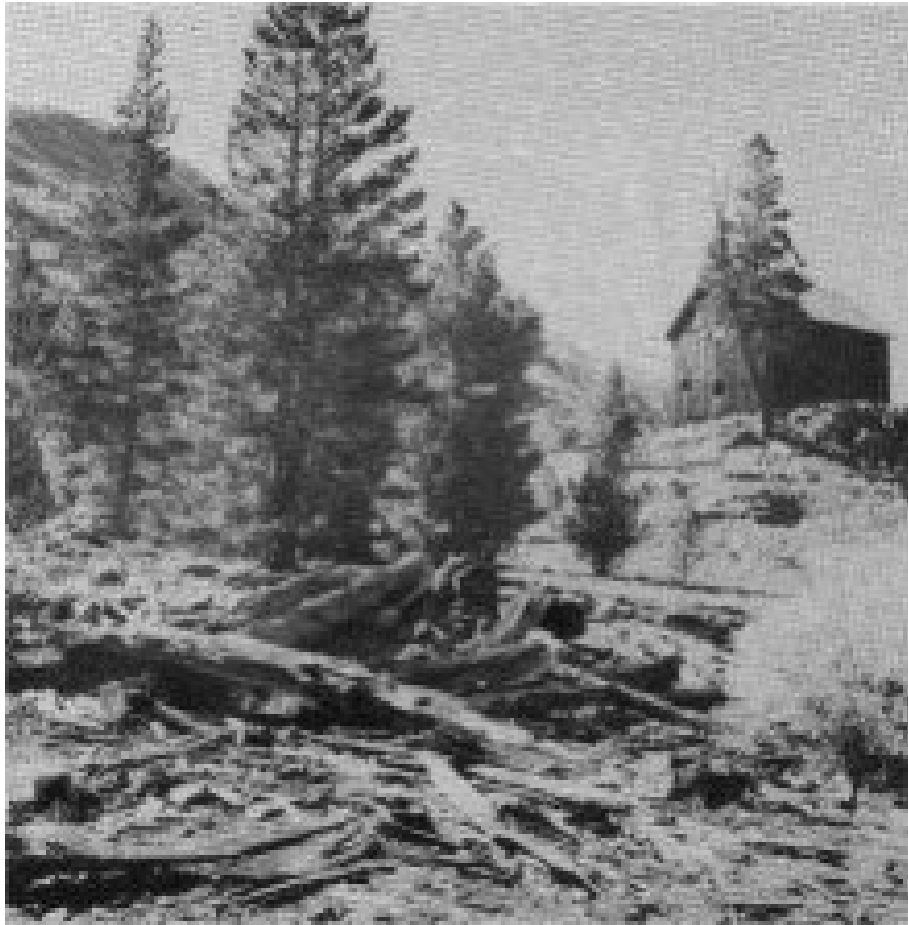
RUINS OF BOARDINGHOUSE BARN AT RIGHT
