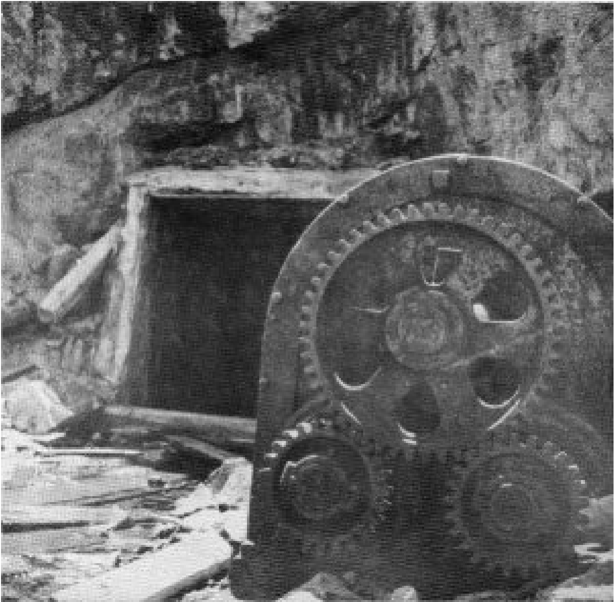
AIR BLOWER AT TUNNEL
