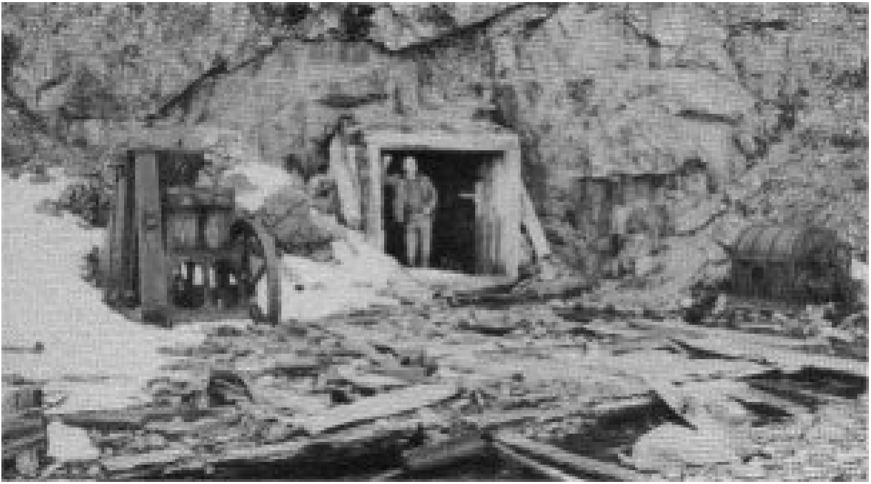
MACHINERY AT TUNNEL (1954)
