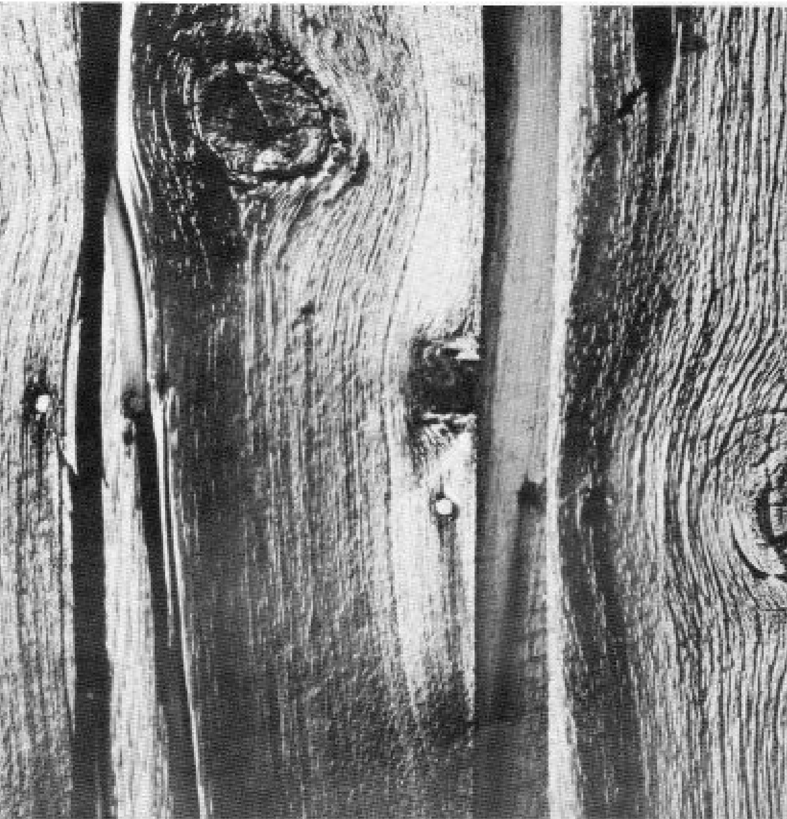
WEATHERED BUILDING, BENNETTVILLE
