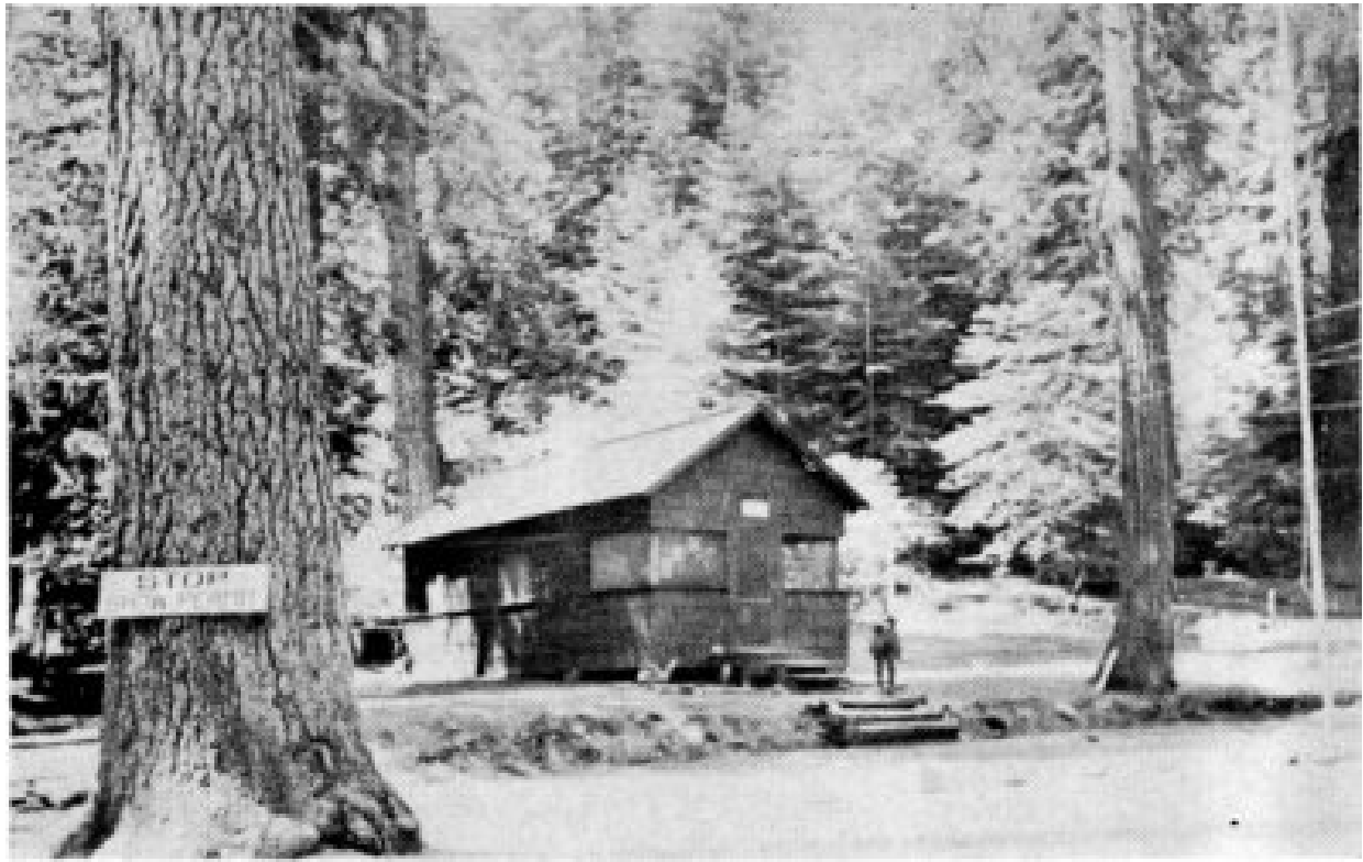
Alder Creek Entrance Station, 1926—Wawona Road
