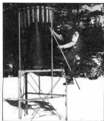
Ranger Bob Johnson measures snow depth and water content at Snow Flat as part of Yosemite snow survey.
