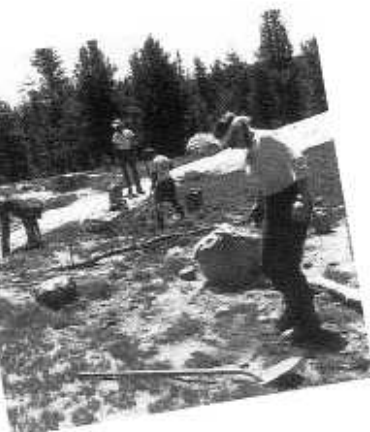
A variety of volunteer help has been of assistance to the skeleton NPS crews responsible for repairing the damaged resources throughout Yosemite.
