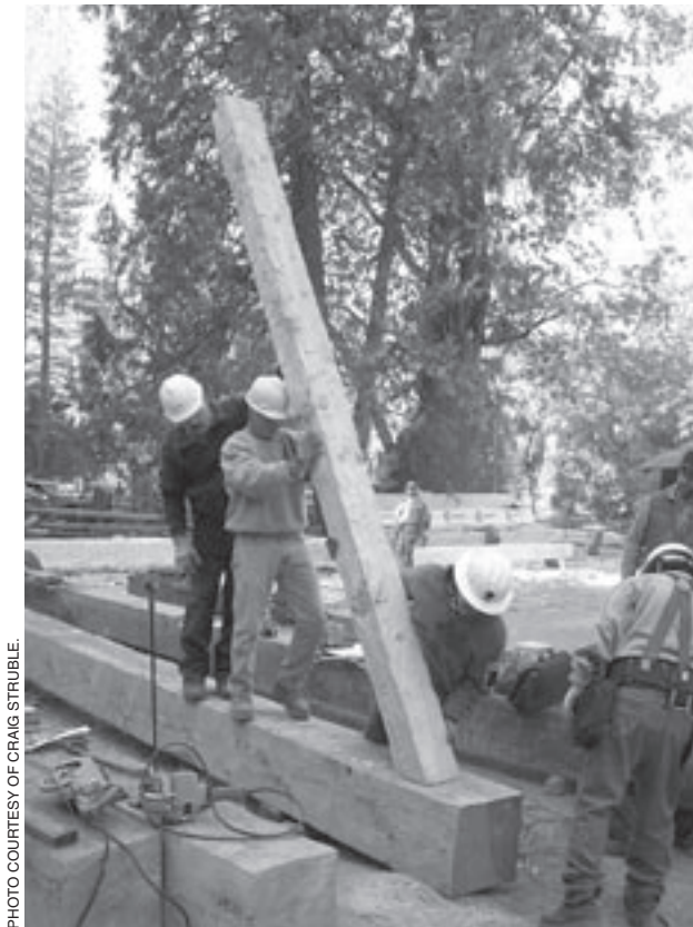
Preservation specialists test fit bridge brace into transverse beam during the 2002-2003 repairs.
