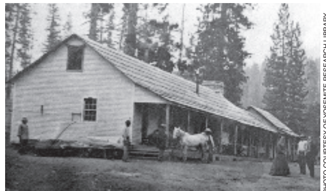
Clark’s Station ca. 1866. The roofline indicates two additions; the chimney may be a remnant from Clark’s original log cabin.
