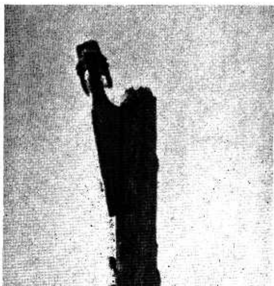
Some of the insulators still cling to the tops of the long-abandoned poles.
