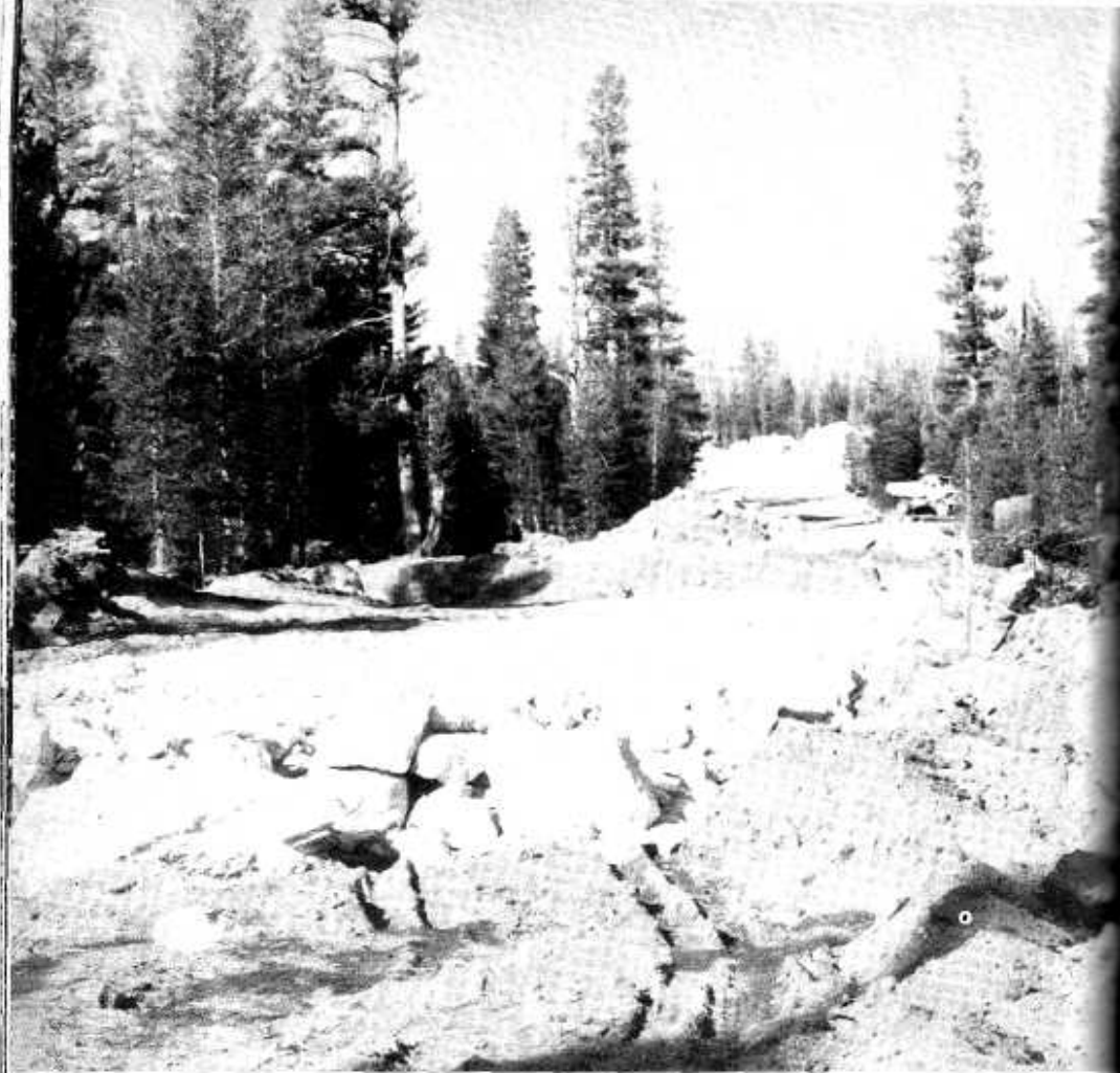
The new Tioga Road is under construction and should be completed by 1961.
