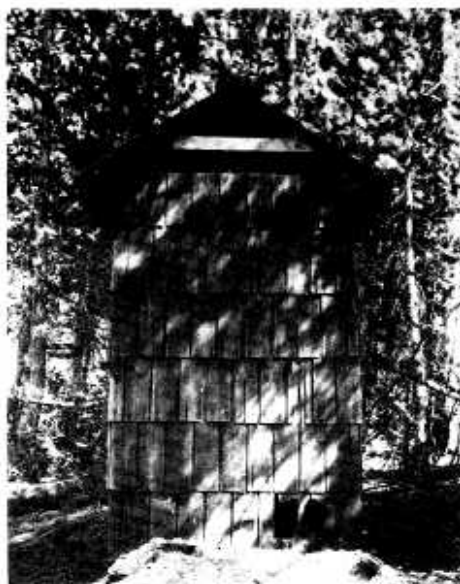
Rundown privies are being replaced.
