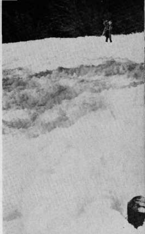
In 1954 Frazil ice covered the bridge — Center post in foreground.
