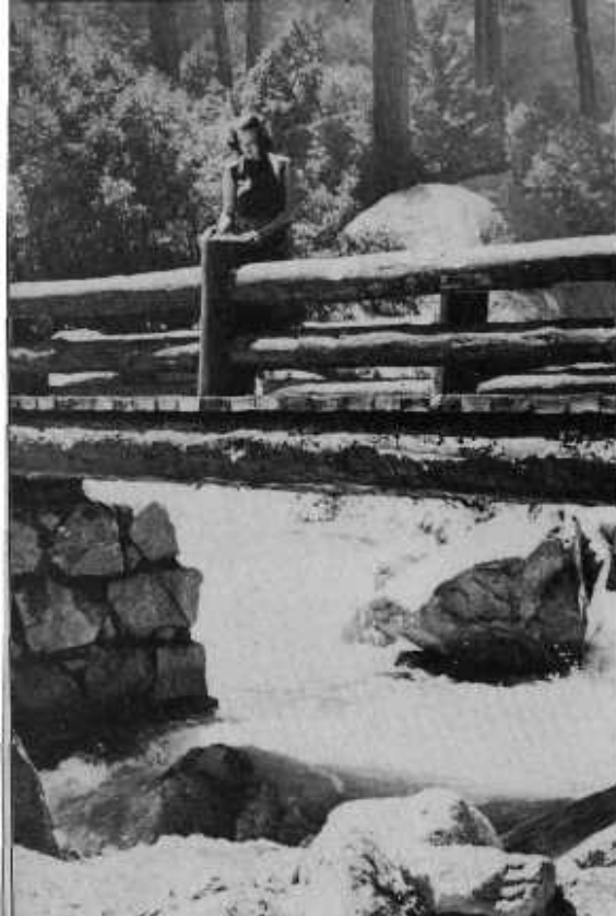
Yosemite Creek Bridge — As visitors usually see it. Note center post.
