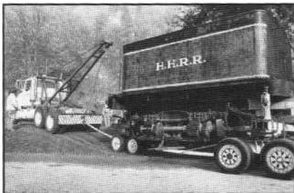
Drive mechanism and water tender from the Shay.
