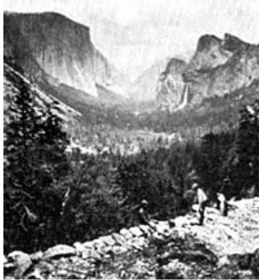
The Gates of the Valley, from Inspiration Point [showing workers constructing the wagon-road]
